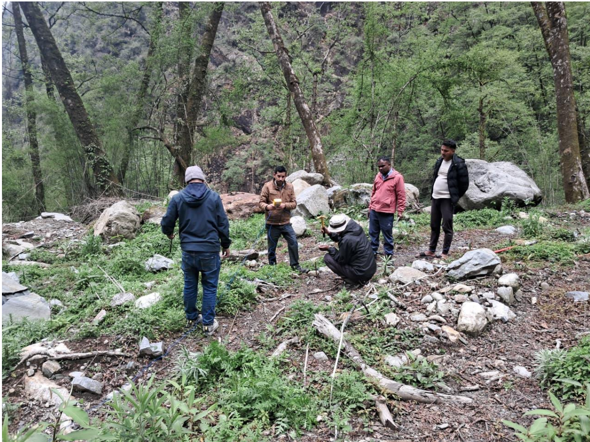
Figure 19: Soil Resistivity test in switchyard area
