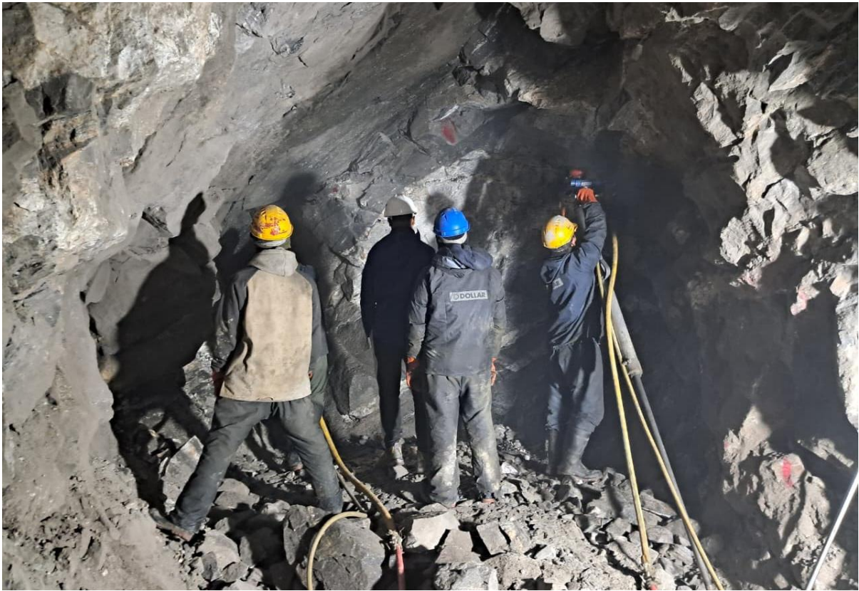
Figure 5: Face drilling in Inlet tunnel at ch 0+038.20m
