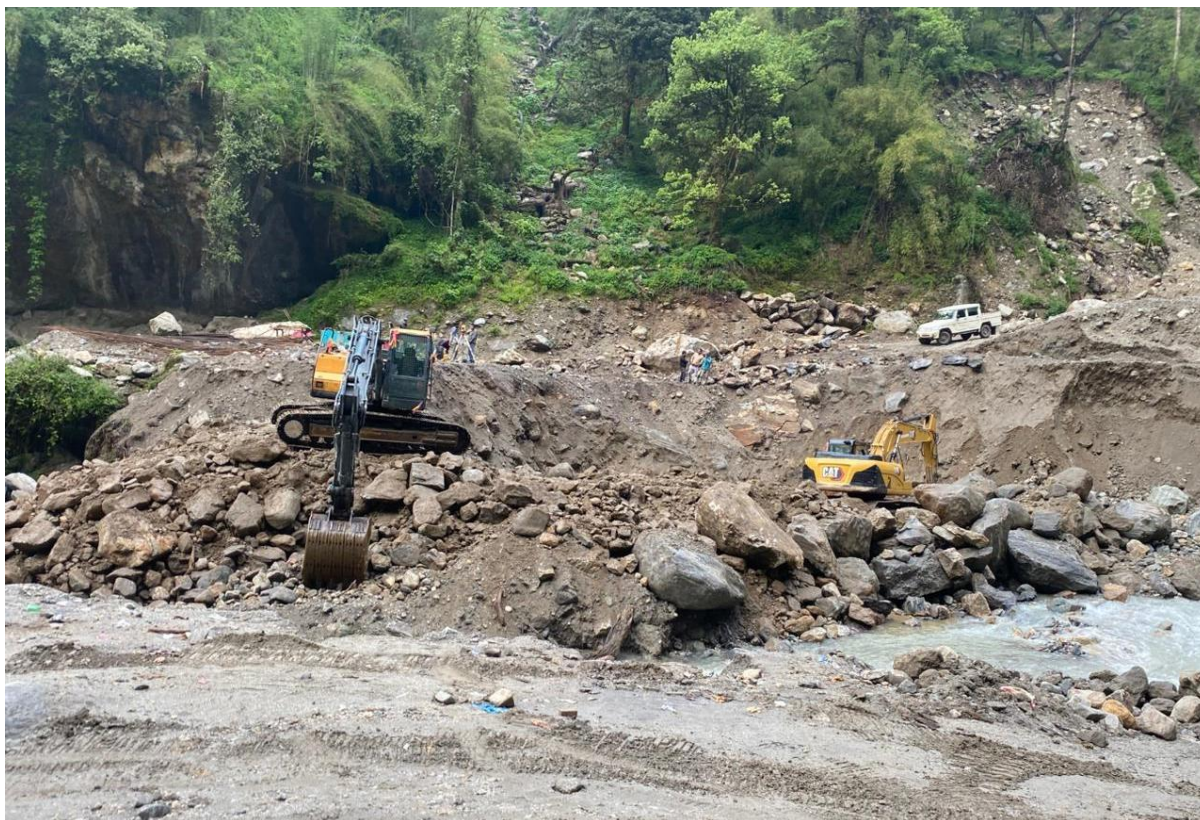
Figure 11: Excavation for bridge right abutment foundation
