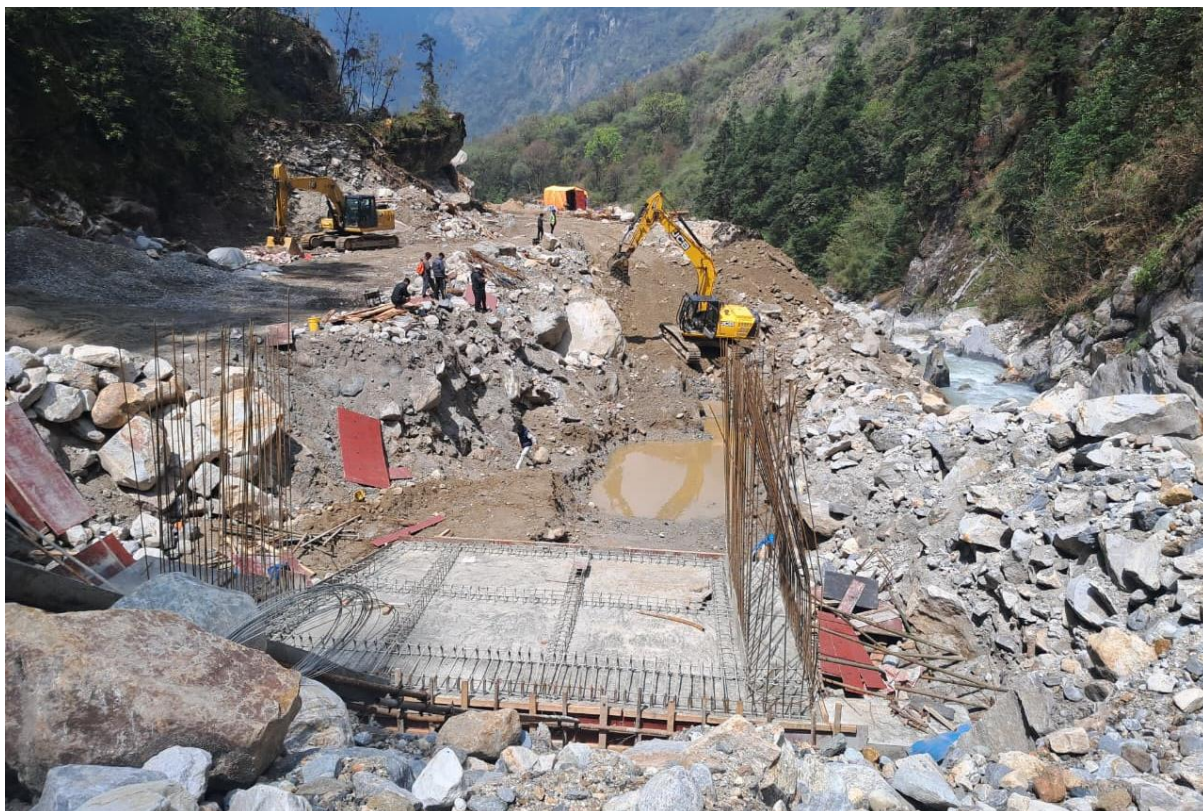
Figure 3: Concreting in Undersluice u/s panel raft and Excavation for Undersluice gated panel
