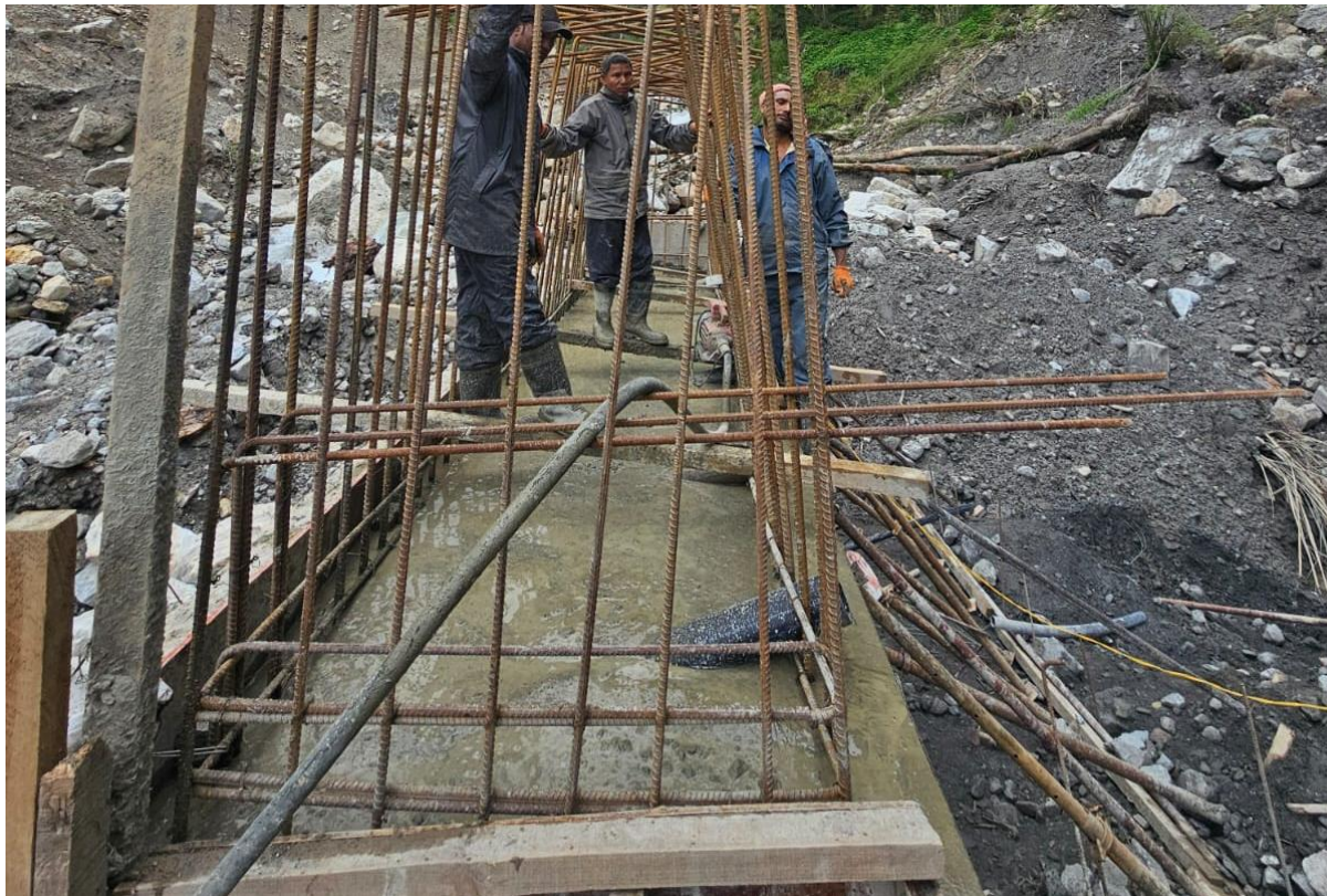
Figure 12: Base concreting in Bridge left abutment
