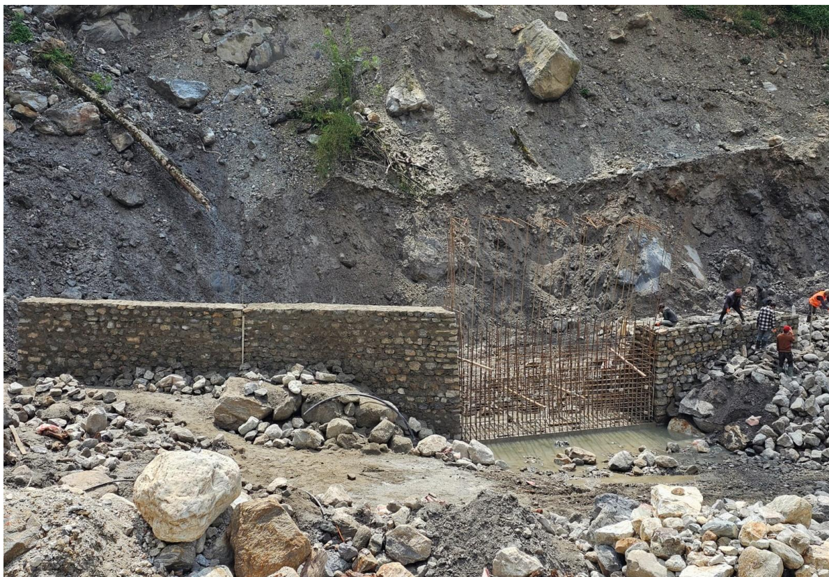
Figure 9: Masonry work in Bridge left abutment
