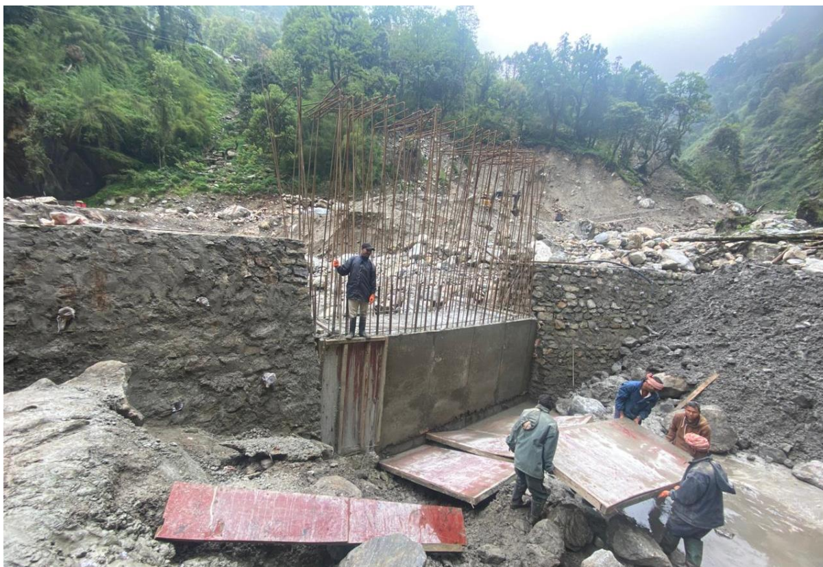
Figure 10: Removing formwork in Bridge left abutment
