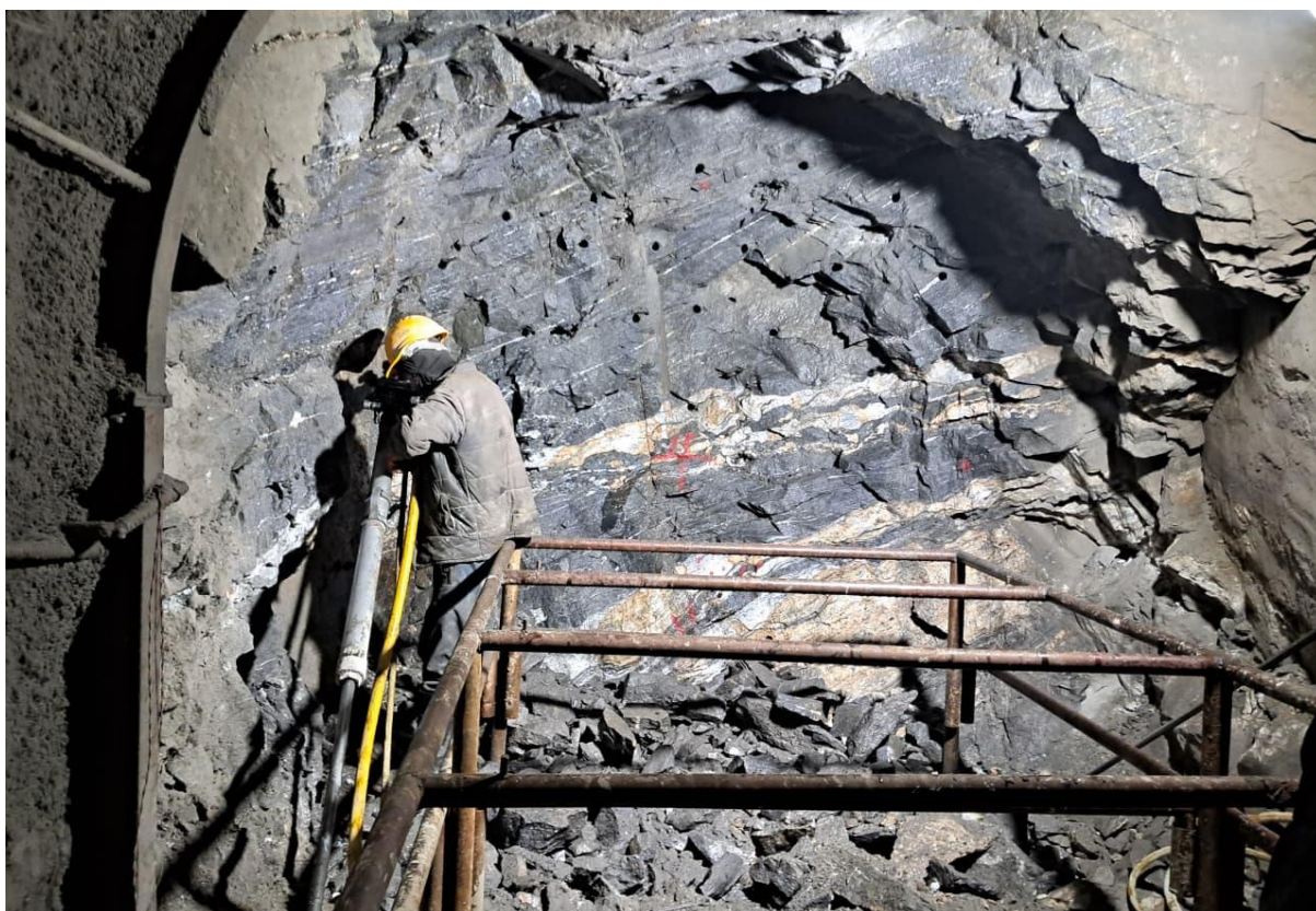
Figure 4: Inlet tunnel face at ch 0+020.90m
