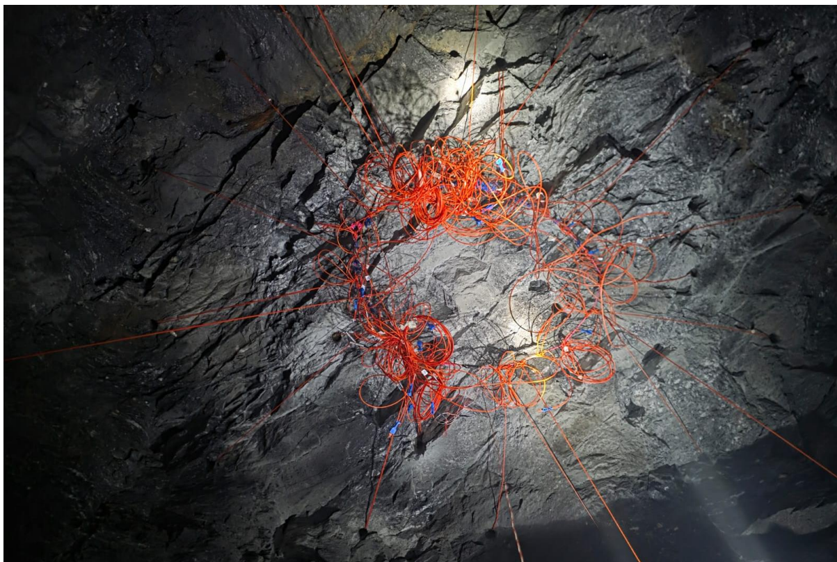
Figure 7: Preparation for blasting in Vertical Shaft tunnel
