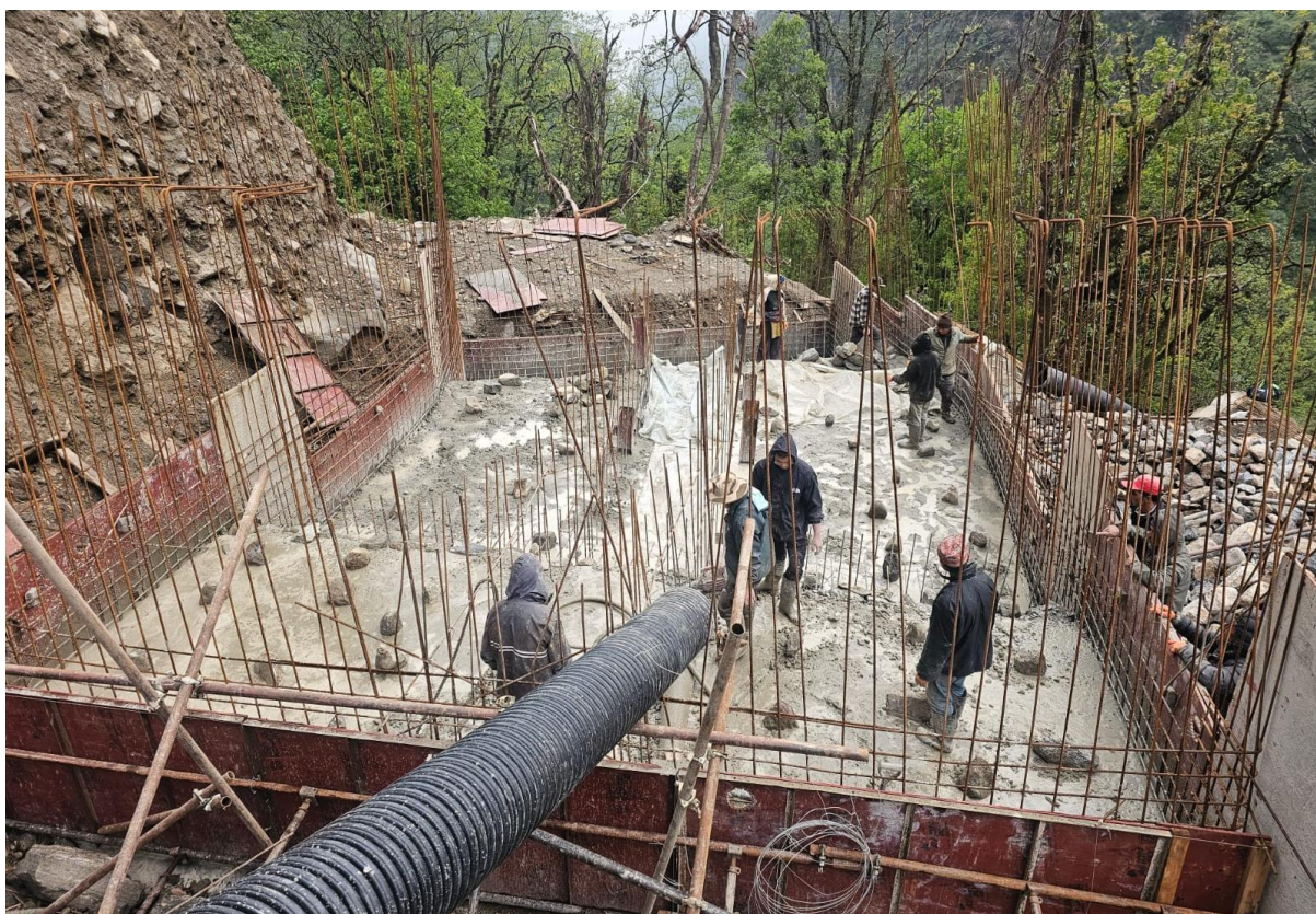
Figure 8: First lift Plum Concrete work in AB-12
