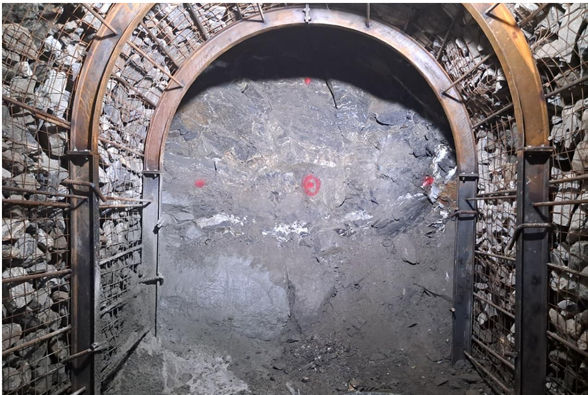
Figure 6: Inlet tunnel face at ch 0+048.90m
