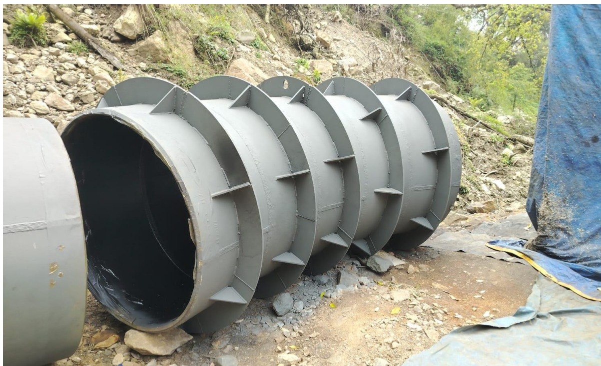
Figure 14: Anchor block 12 bend pipe after painting
