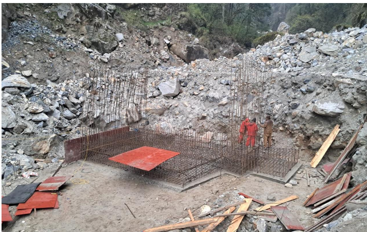
Figure 2: Rebar and formworks in Undersluice u/s cutoff in Headworks
