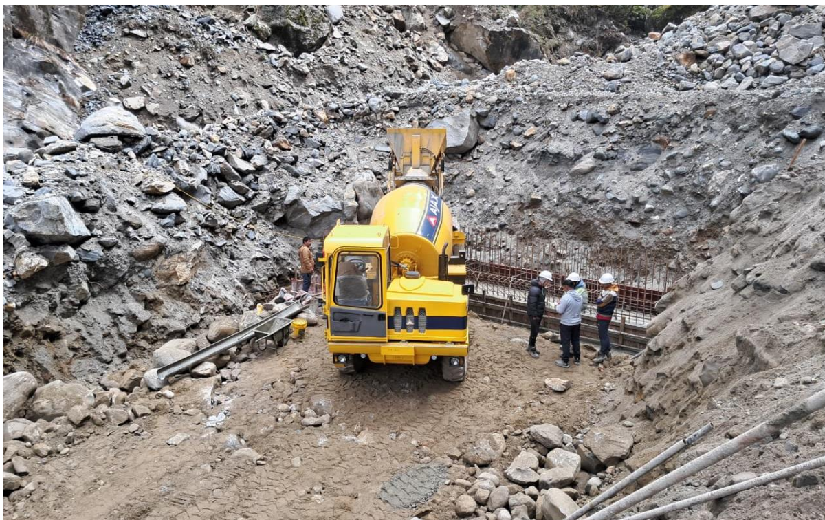
Figure 1: Concrete pouring by SLM in Undersluice u/s cutoff wall
