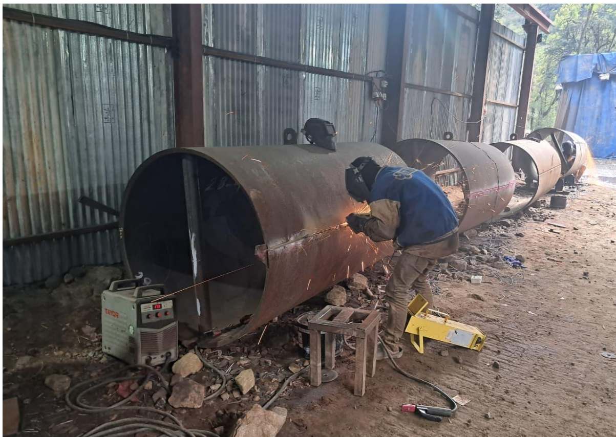
Figure 13: Grinding work in pipe
